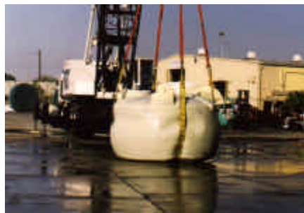
Figure 3 Crosslinked Tank No Failure
